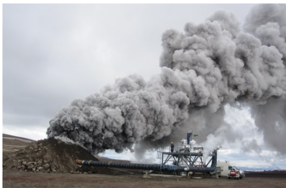
Figure 1: Flow test of IDDP-1. For the first hours during the flow test the steam is grey colored due to corrosion products.
